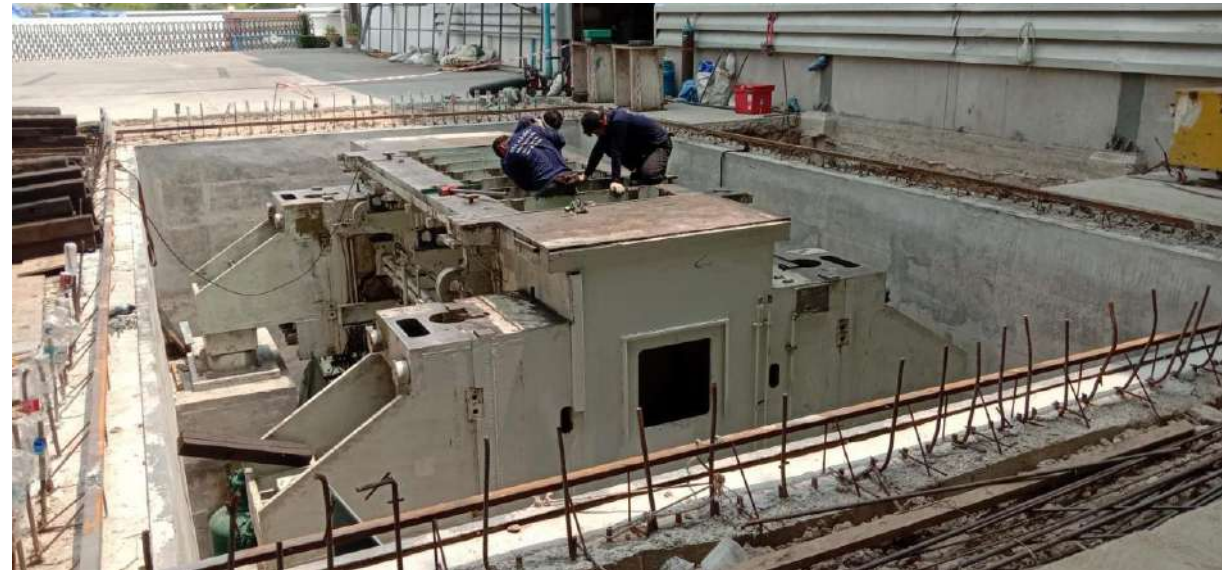
Foundation Pit for Komatsu 1700 ton Press
