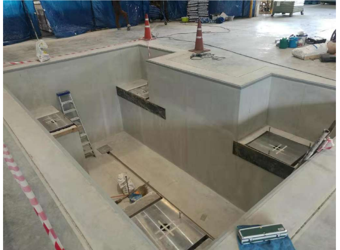
Foundation Pit for Seyi 600 ton Press
