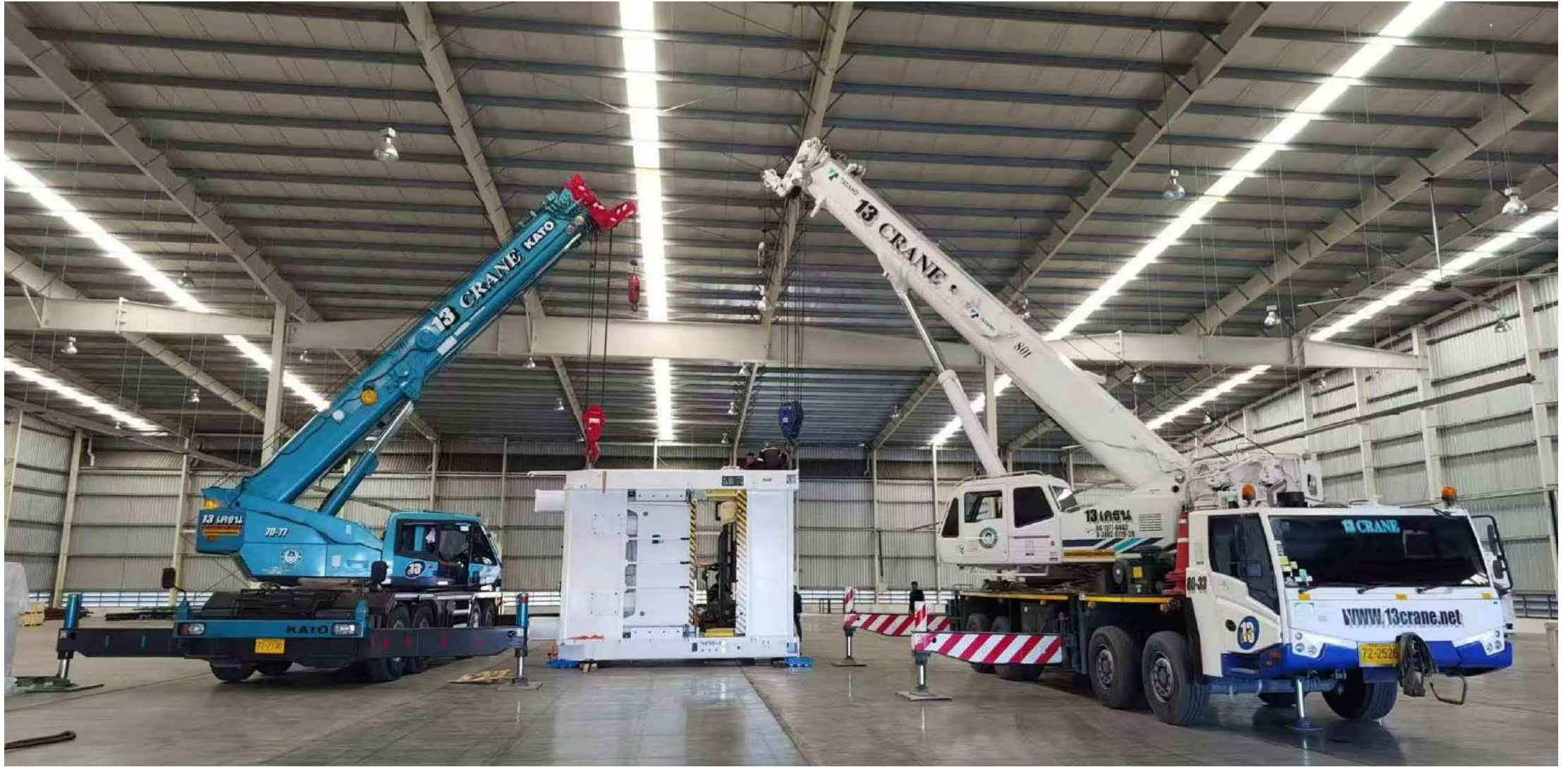
Installation of 500 Ton Yangli Press. Machine Weight: 65 ton
